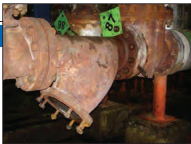
FIGURE 10. The “Y” filters were inspected
