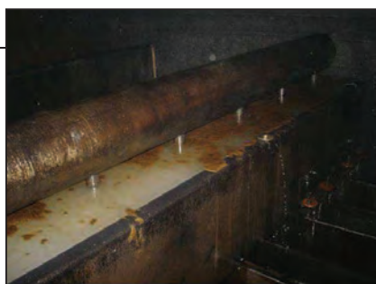
FIGURE 7. This blockage required that the distributor be dismantled and cleaned
